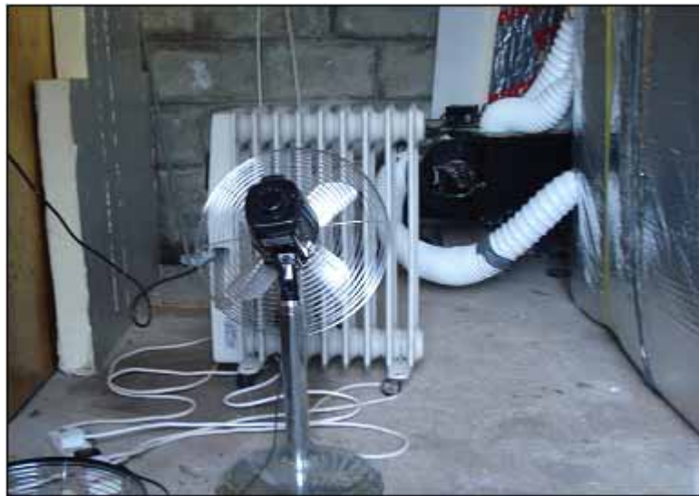
Figure 5.21: Fan and Heater in Place
