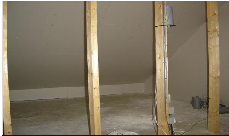
Figure 2.12: Plasterboard Lining on inside of Test Structures [40]
