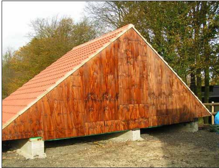
Figure 2.10: Outside View of Finished Test Structure, High-Wycombe [40]
