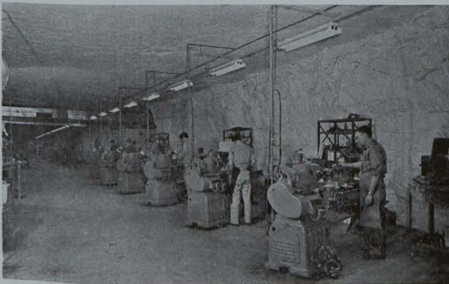
One of the workshop-tunnels in the air-conditioned underground factory of the Brunson Instrument Company.
