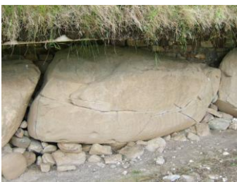
Figure 4. Shattered kerb stone at Knowth Brú na Bóinne (C. Daly 2009)
