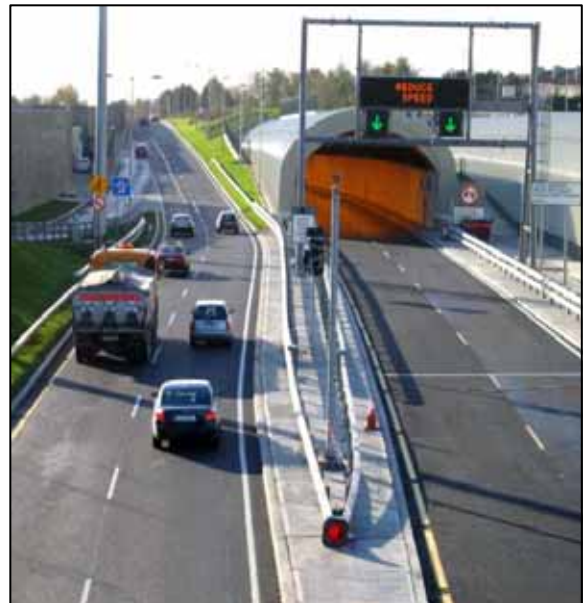
Figure 1.4. Photograph showing the Dublin port access tunnel
