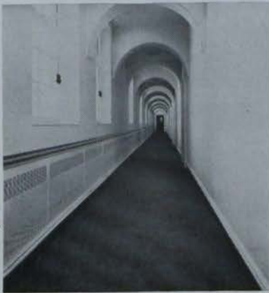
Dunham-Bush multi-purpose converters are pictured in a continuous modular installation.
