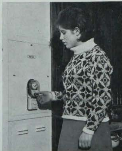
By operating a clock control panel on the face of the G 4501 the householder can pre-set the heating programme for the day.
