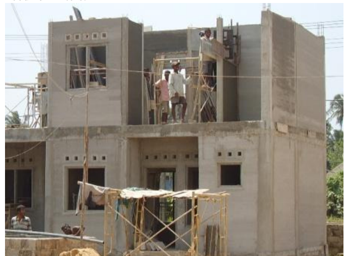
Fig 4 Shows Slip Form wall construction with team of three unskilled labourers
