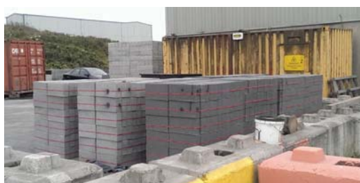
Figure 1b. Block stacks on site.
