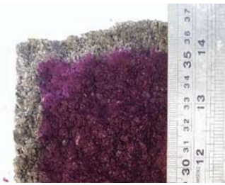
Figure 3. Measuring depth of carbonation.
