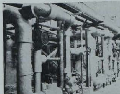
The Esso petro-chemical plant goes on steam at Stenungsund, Sweden. The insulation of the refrigeration system was carried out with Newallite Polyurethane.
