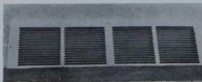
Shown here is the C55 Hiboy, fully automatic Kresky-fired warm air heater, and below is one of the low wall return air grilles featured in the Malahide installation reported on page eleven.
