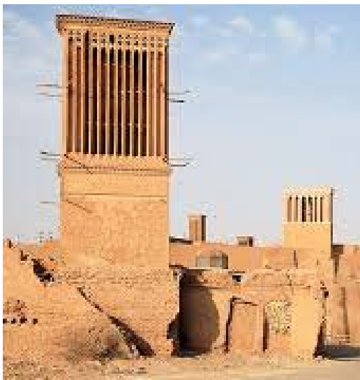
Figure 16: Badgir, wind scoop and exhaust.
