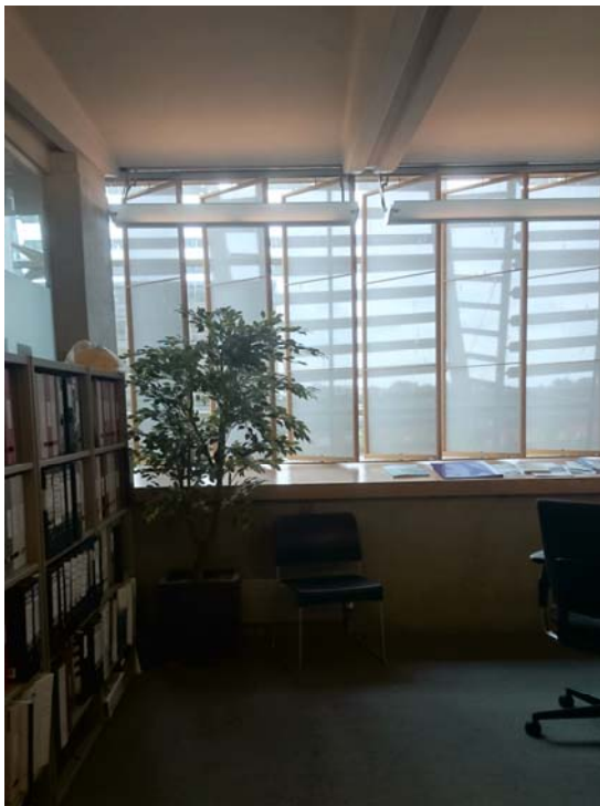
Figure 68: office showing exposed thermal mass of the ceiling slab
