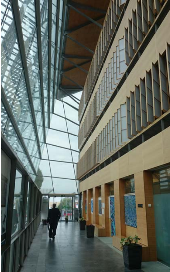
Figure 61: internal view of atrium showing manually operated glare control blinds on the right
