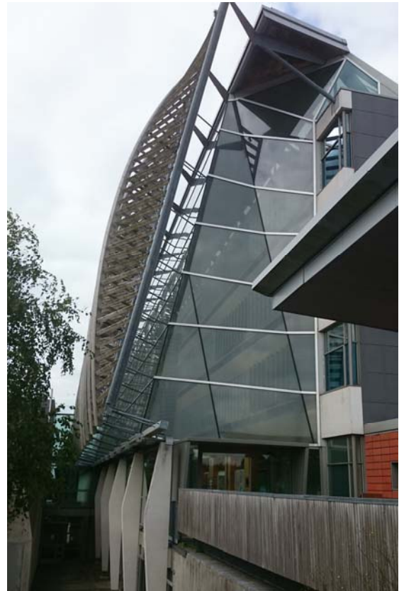
Figure 60: south east end to atrium
