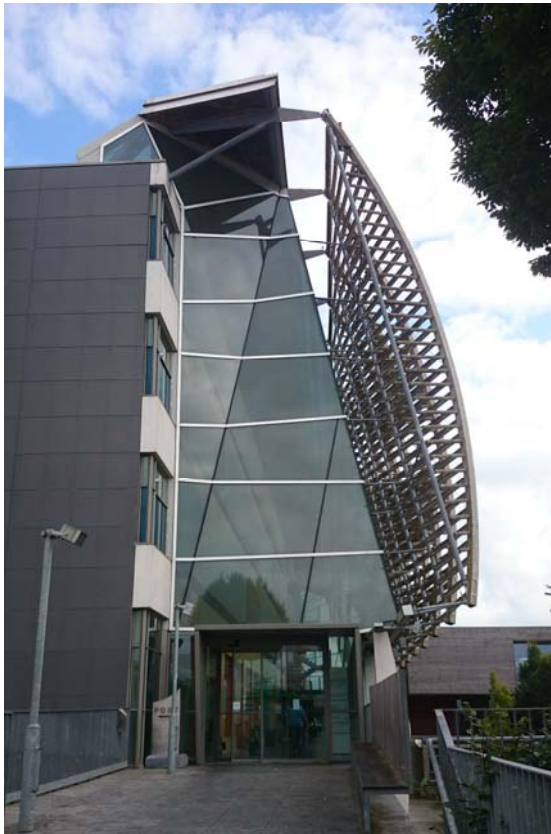
Figure 59: north west end to atrium
