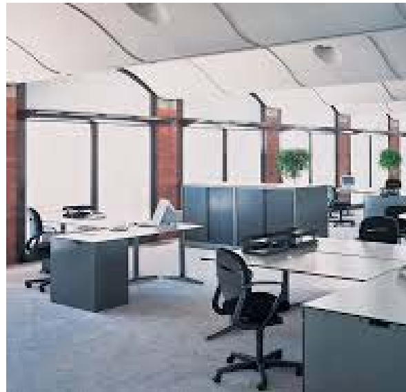
Figure 32: Inland Revenue Centre, internal view showing sinusoidal ceiling to expose thermal mass (Hopkins Associates)
