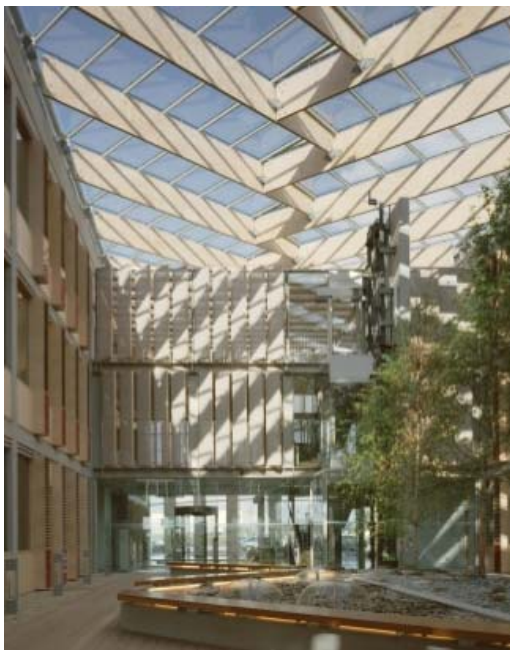
Figure 70: SAP Building, Galway – showing the internal atrium – (Bucholz-McEvoy Architects)
