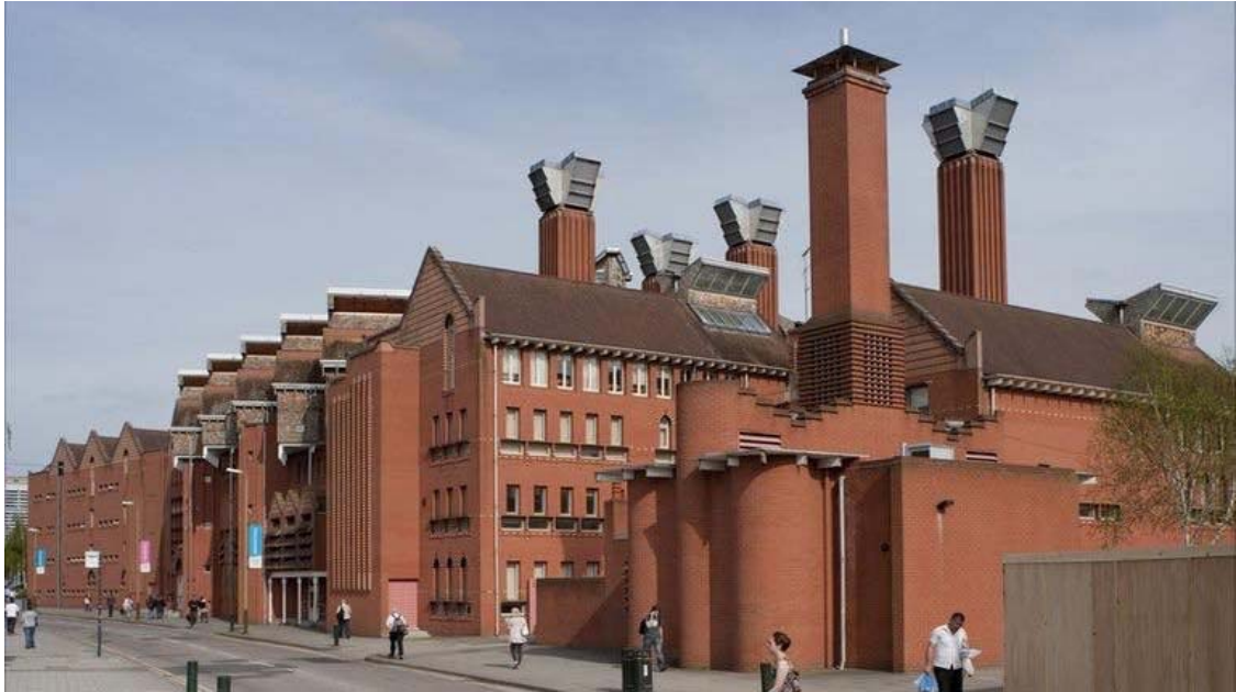
Figure 50: Queens Building, ‘edge in – centre out’ ventilation – inlet vents visible on street elevation and chimney stacks outlets - Short Ford Associates
