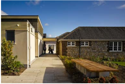
Figure 28: Bench topped air inlet to earth tubes, Airfield Estate, (Solearth Architecture)
