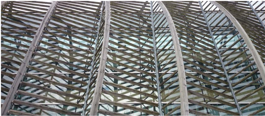
Figure 55: detail of timber brise-soleil to atrium facade
