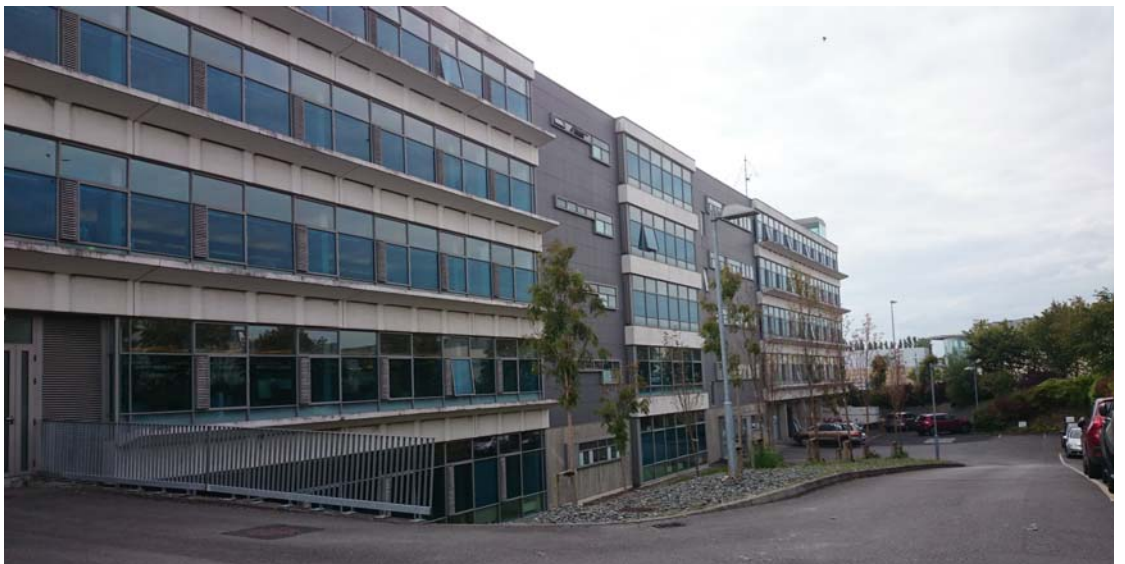
Figure 53: north east façade showing air intakes incorporated into the glazing system
