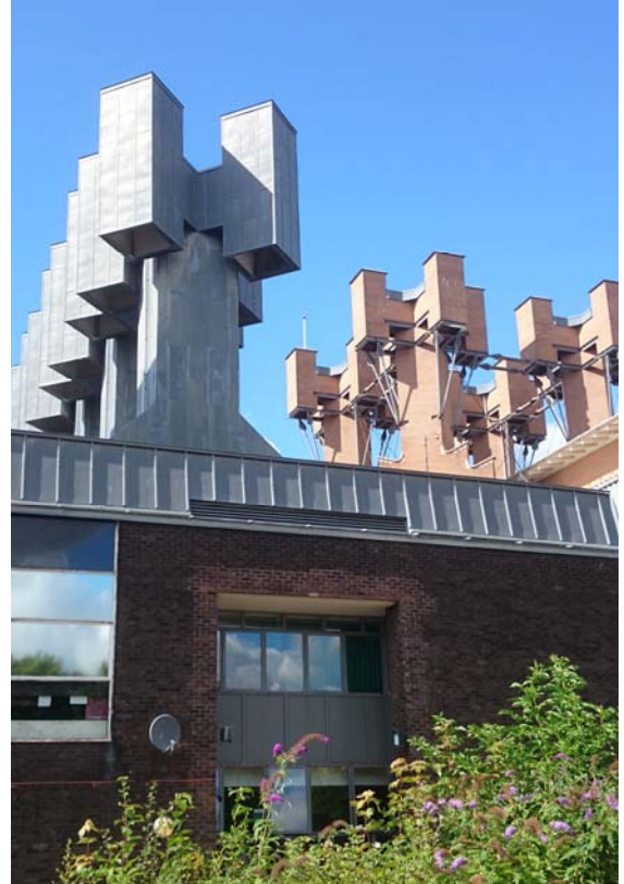
Figure 93: insulated zinc-clad stacks to main theatre
