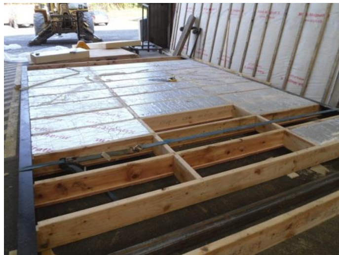
Figure 48: Image of floor slab during pre-fabrication
