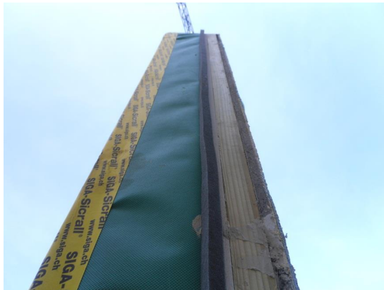
Figure 71: Image of end detail of Wall 1 before being positioned. The external breather membrane (green) is wrapped and taped on the inside of the wall (yellow) before the addition of the Compriband strip
