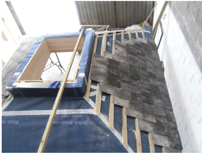
Figure 51: Image of roof section during pre-fabrication
