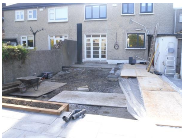
Figure 86 Images showing footprint of building before installation and positioning of ground floor slab
