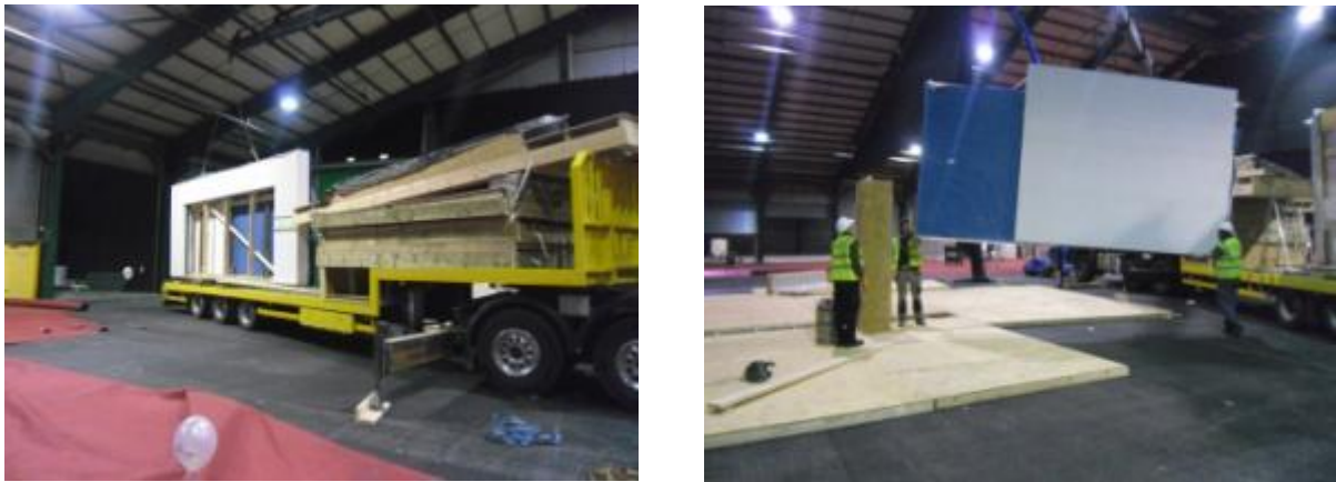
Figure 58: Images of wall and roof panels on flat-bed truck and being lowered into position
