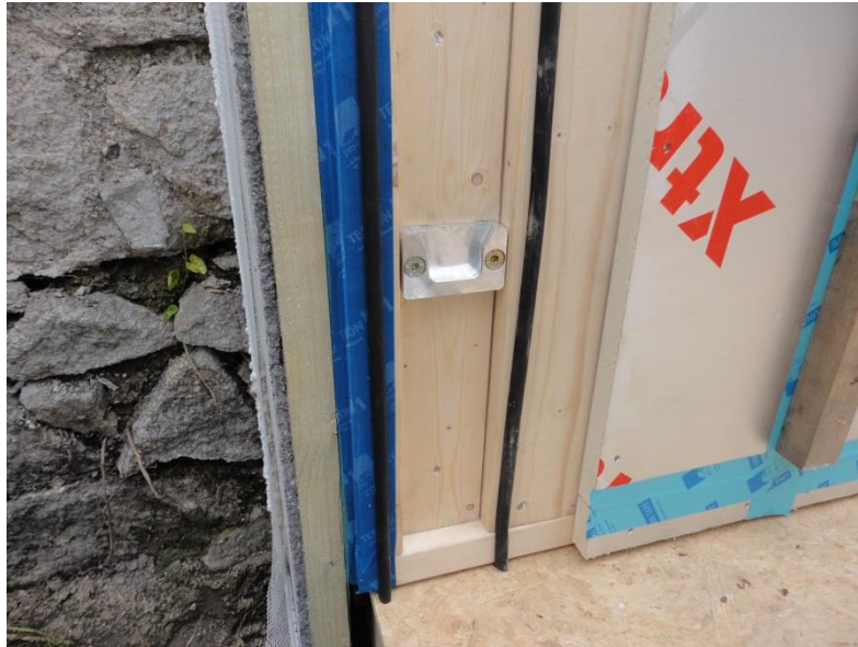
Figure 78: Bituminous layer with EPDM sealant between new and old building
