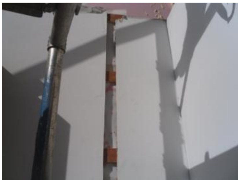
Figure 52: Joint between the 100mm wall panels after positioning
