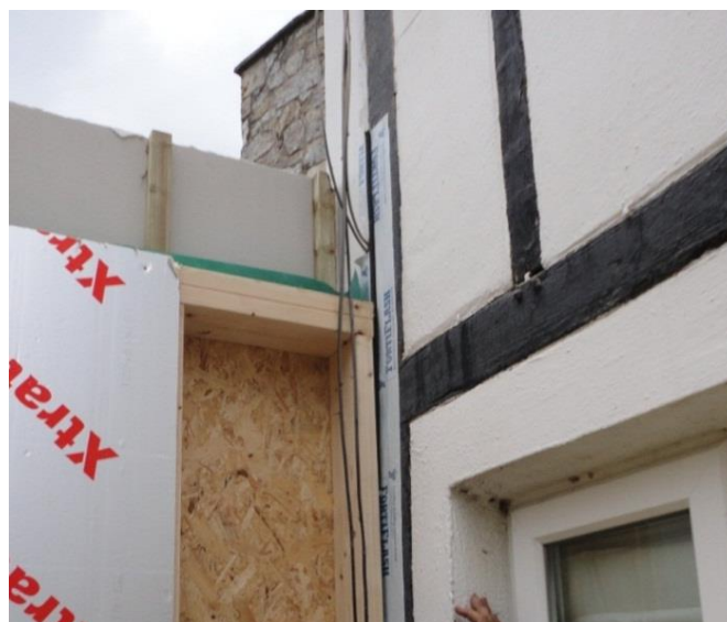
Figure 79: Image of connector and EPDM rubber strips in position prior to joining Wall 1 and 2
