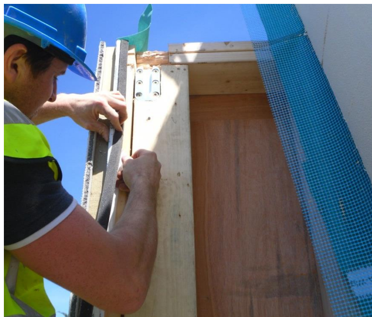
Figure 72: Installation of Compriband tape after the external breather membrane has been taped to the end stud
