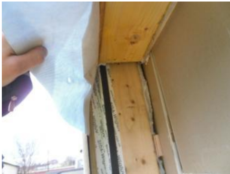
Figure 54: Image of final panel sliding into position (Compriband tape visible)
