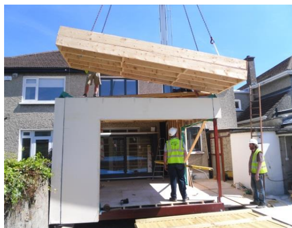
Figure 69: Images showing the fall in each roof panel and also installation of the panels on-site
