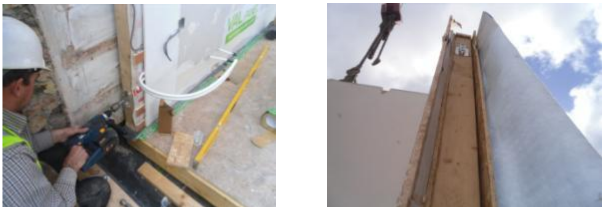
Figure 53: Application of SHERPA connectors to positioned wall
