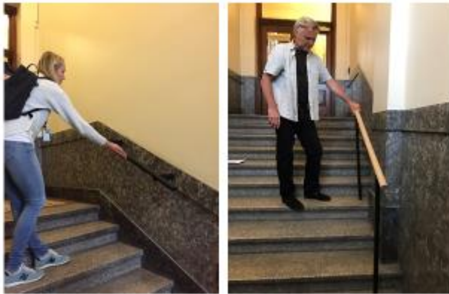
Figur 8. Norwegian High Court. Testing out different types of new handrails. Photo: Statsbygg
