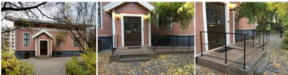
Figure 7. Grotten 1841. Honorary house. Statsbygg also maintain some honorary housing. New ramp leading up to the main entrance. Photo: Statsbygg
