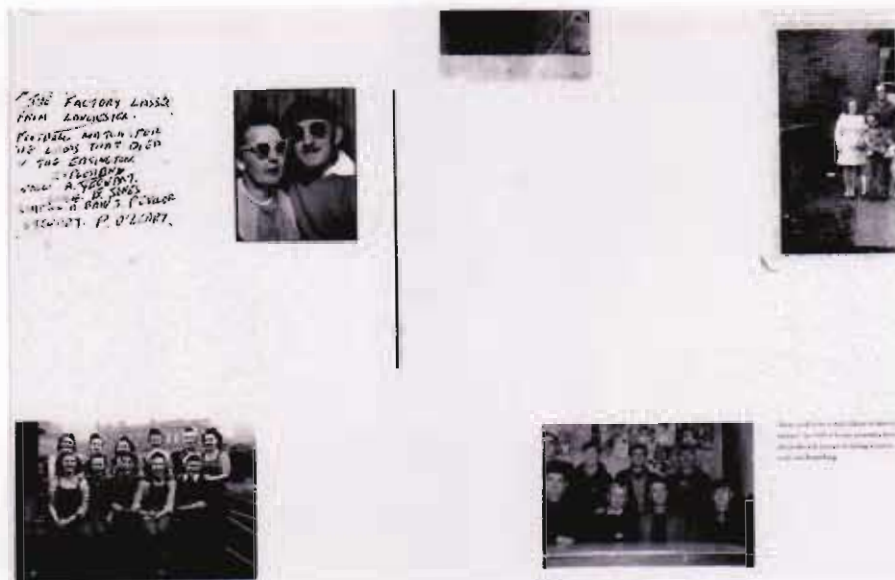
Figure 3.2; from Steelworks , Julian Germain
