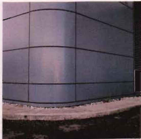
Figure 2.18; unused from Building 2 (exterior) HP, August 2003
