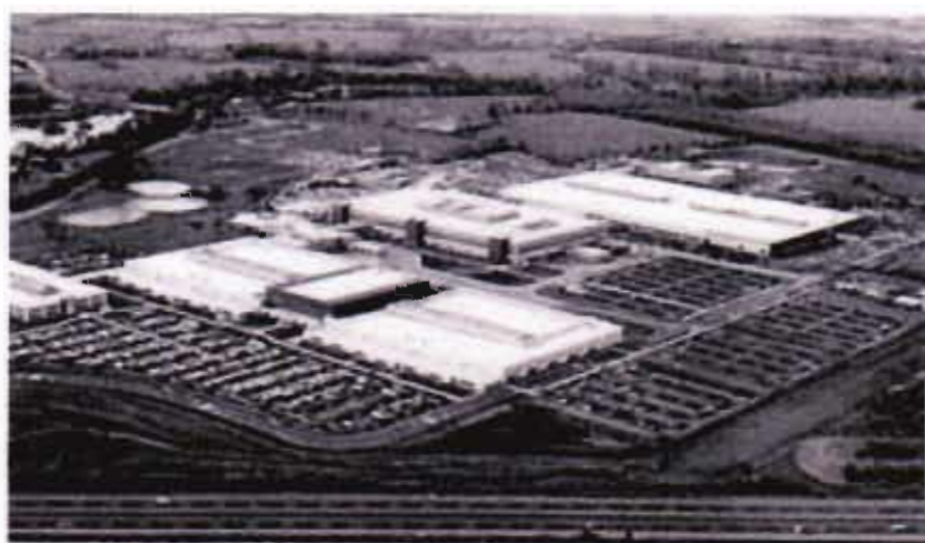
Figure 1.5; Hewlett-Packard (Manufacturing Limited) Liffey Park Technology Campus, Barnhall, Leixlip, County Kildare (source: HP)
