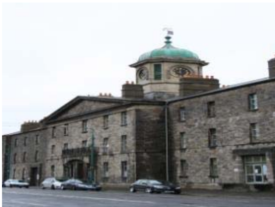
Fig 2: Clocktower Building, Grangegorman (DIT photo)
