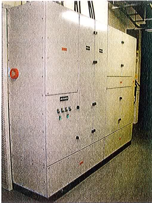
Balancer Switchboard
