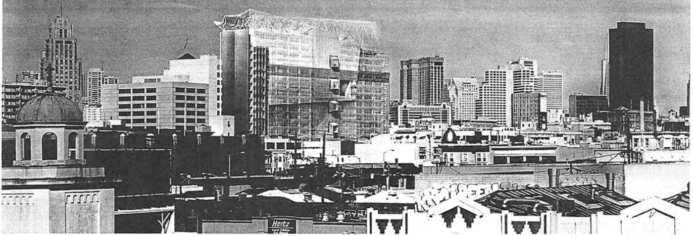
San Francisco Federal Office Building, Morphosis/Smith Group
