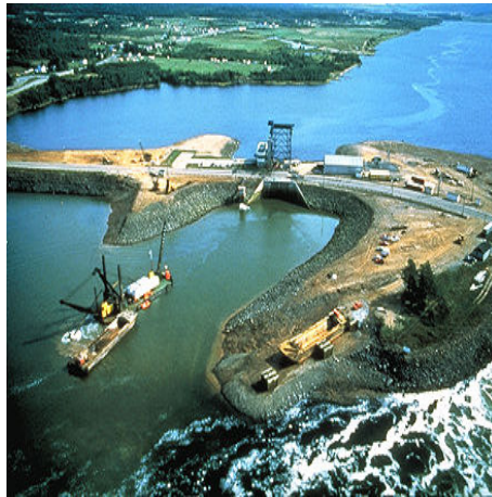
Figure 3. The Annapolis Tidal Power Facility[23]
