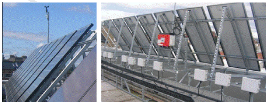
Fig. 1. The PV system installation.
