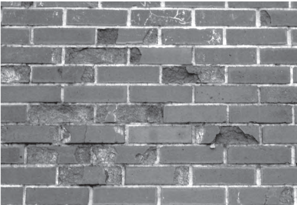
Figure 10.3. Surface Deterioration from Sub-freezing Consistently Moist Brick.
