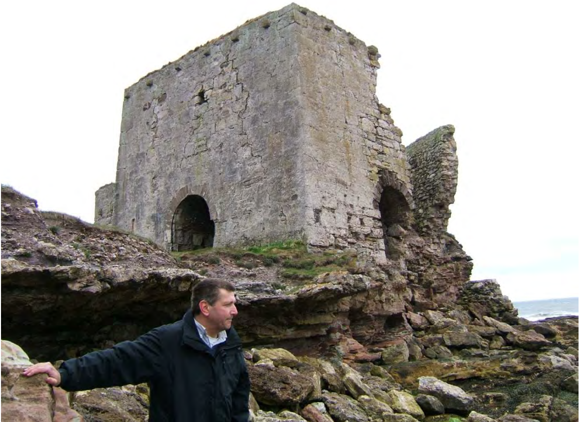
Figure 5.11. Boddin Limekiln showing undercutting and collapse due to wave action, Tom Dawson in foreground, April 2012
