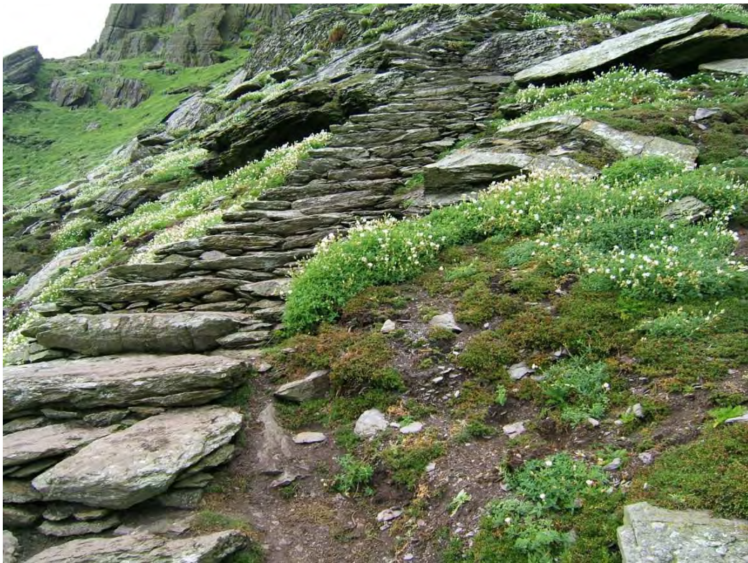
Figure 7.4. Vegetation and soil erosion due to visitor traffic on steps to monastery August 2010
