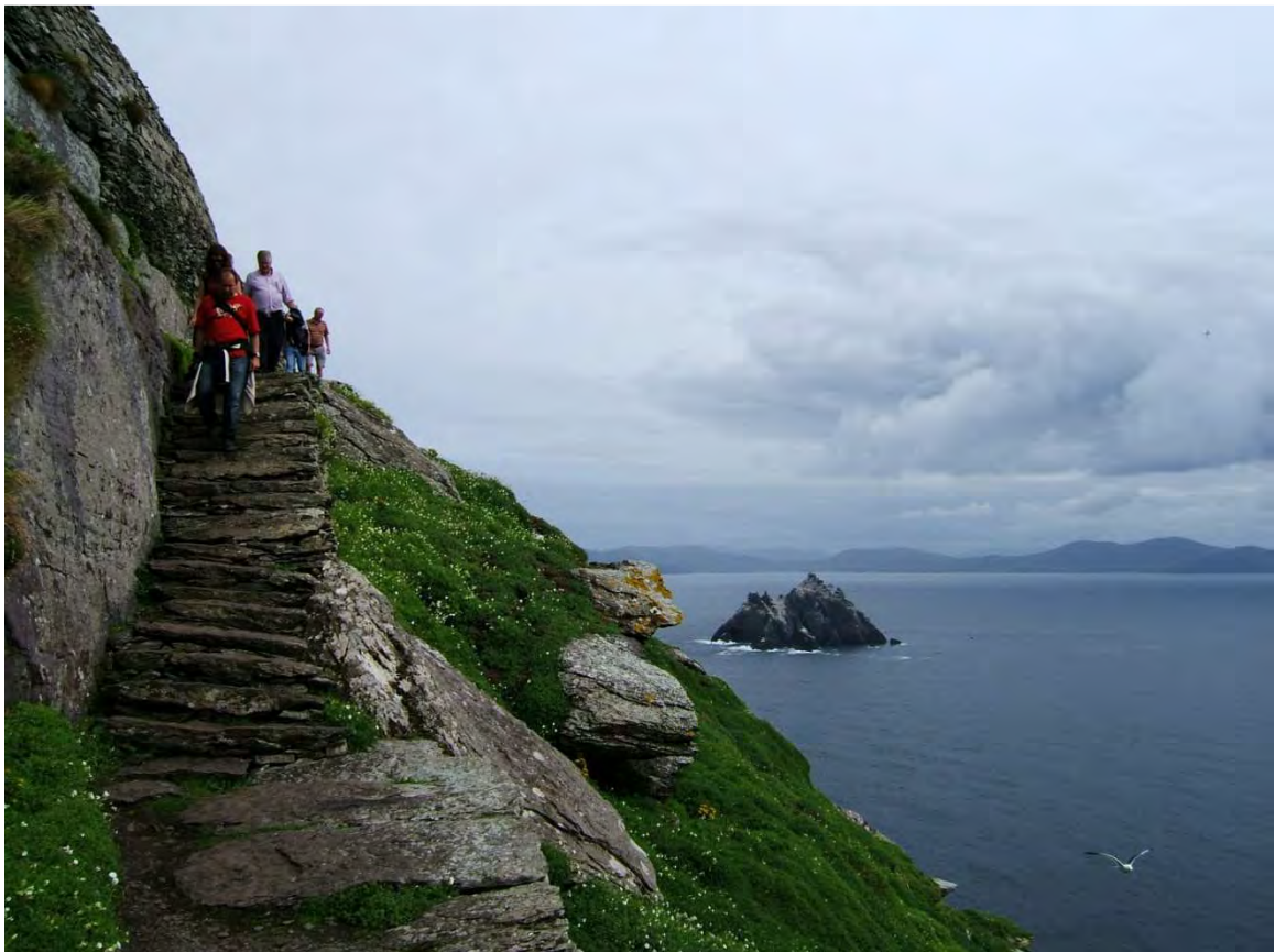
Figure 7.3. Steep topography and dry stone Medieval staircases that characterise Skellig Michael, August 2010
