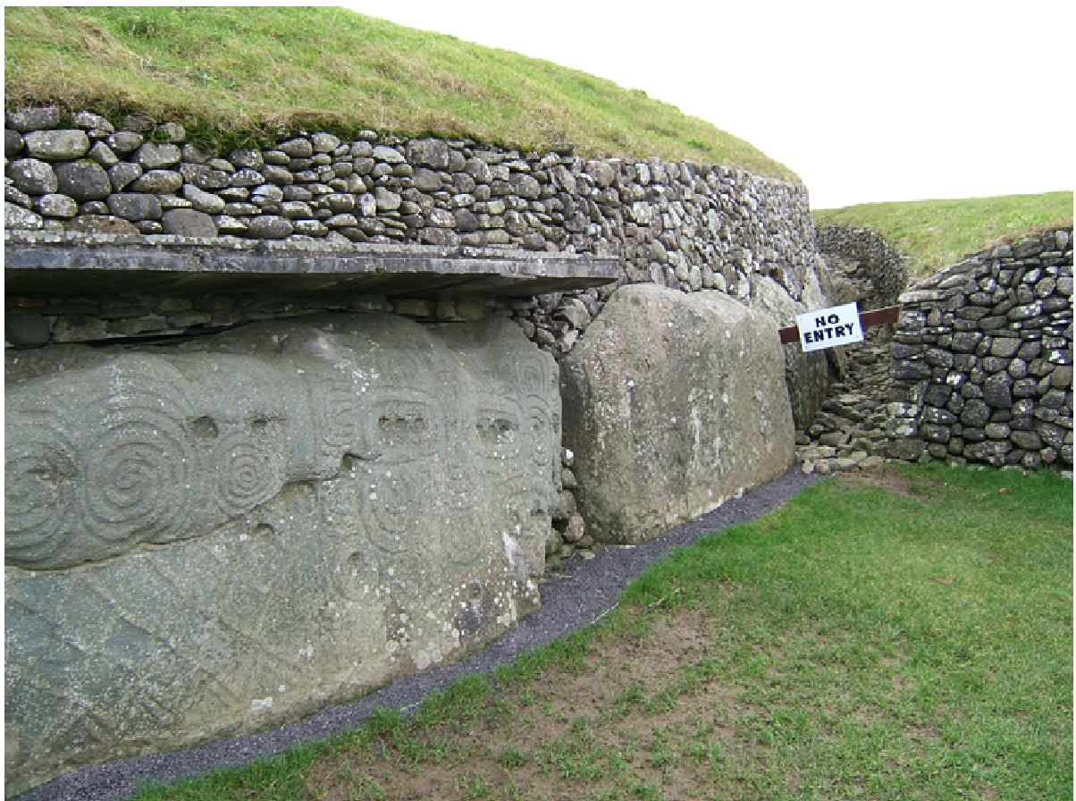
Figure 8.11. Kerbstones at Newgrange south-east side: Excavated area in foreground with cantilevered shelter; unexcavated area behind with stone faced concrete revetments on both the mound and ditch (cut through cairn collapse) (April 2009)
