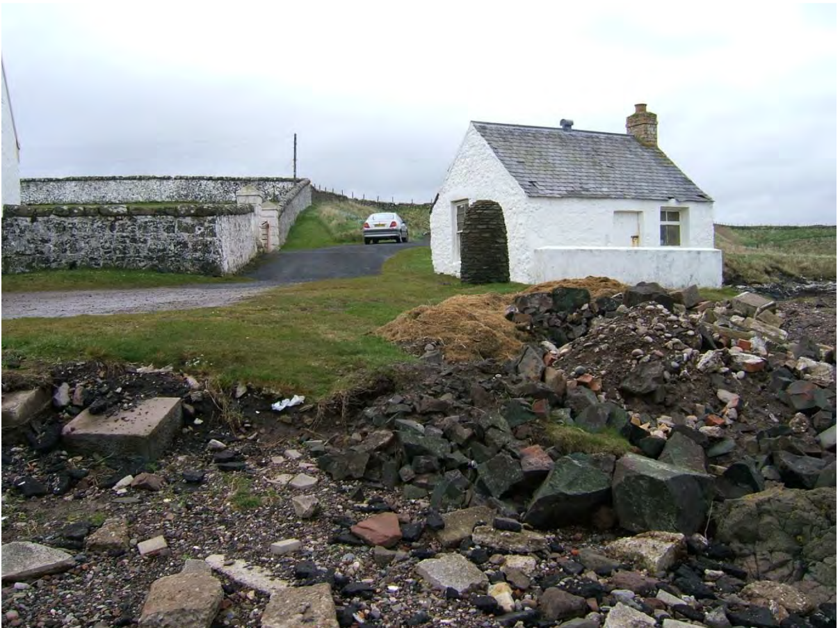
Figure 5.13. Ad hoc attempts to prevent erosion occur at local level regardless of Shoreline Management Plans e.g. the deposition of building rubble and garden waste by owners of Scurdie Ness Lighthouse, April 2012
