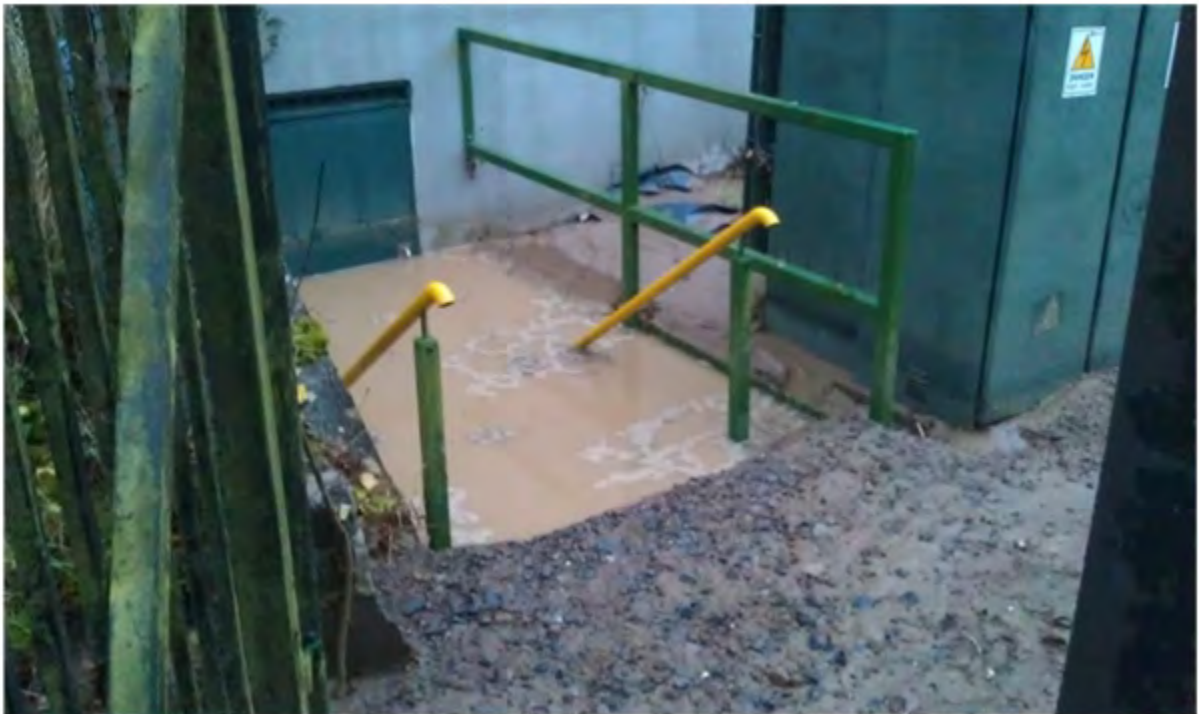
Figure 8.8. Visitor Centre treatment plant flooded with soil and potatoes after heavy rain in October 2011 (Tuffy 2011)
