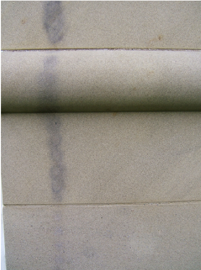
Figure 5.5. Staining from electrical resistance tomography, February 2012
