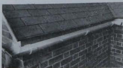
● Section of Osma rainwater system
