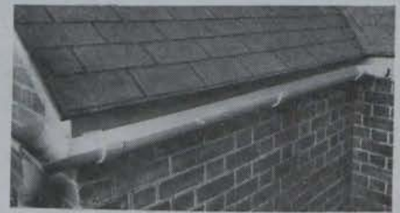
● Section of Osma rainwater system.
