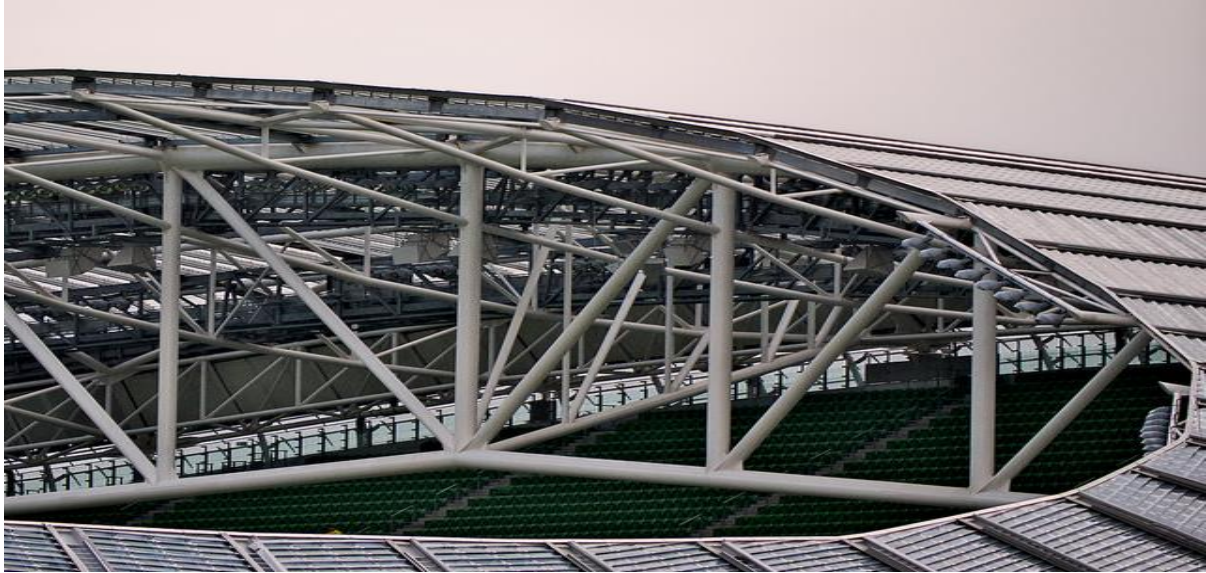
Fig 15 – Roof steel on the Aviva Stadium (Source: www.flickr.com )
