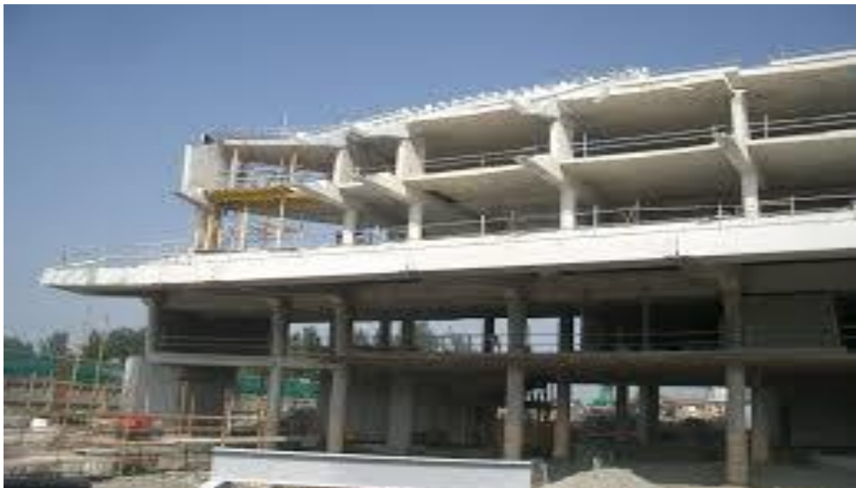
Fig 14 - Precast Concrete frame construction (source: www.patkirwan.ie )
