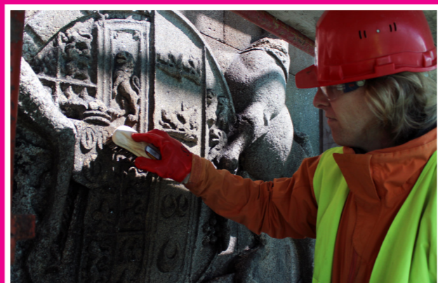
Coat of arms being cleaned on the Lower House
