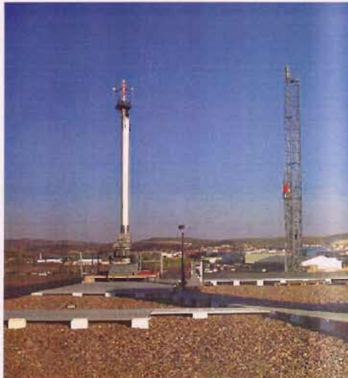
Fig. A5.2: Free space elevated antenna range
