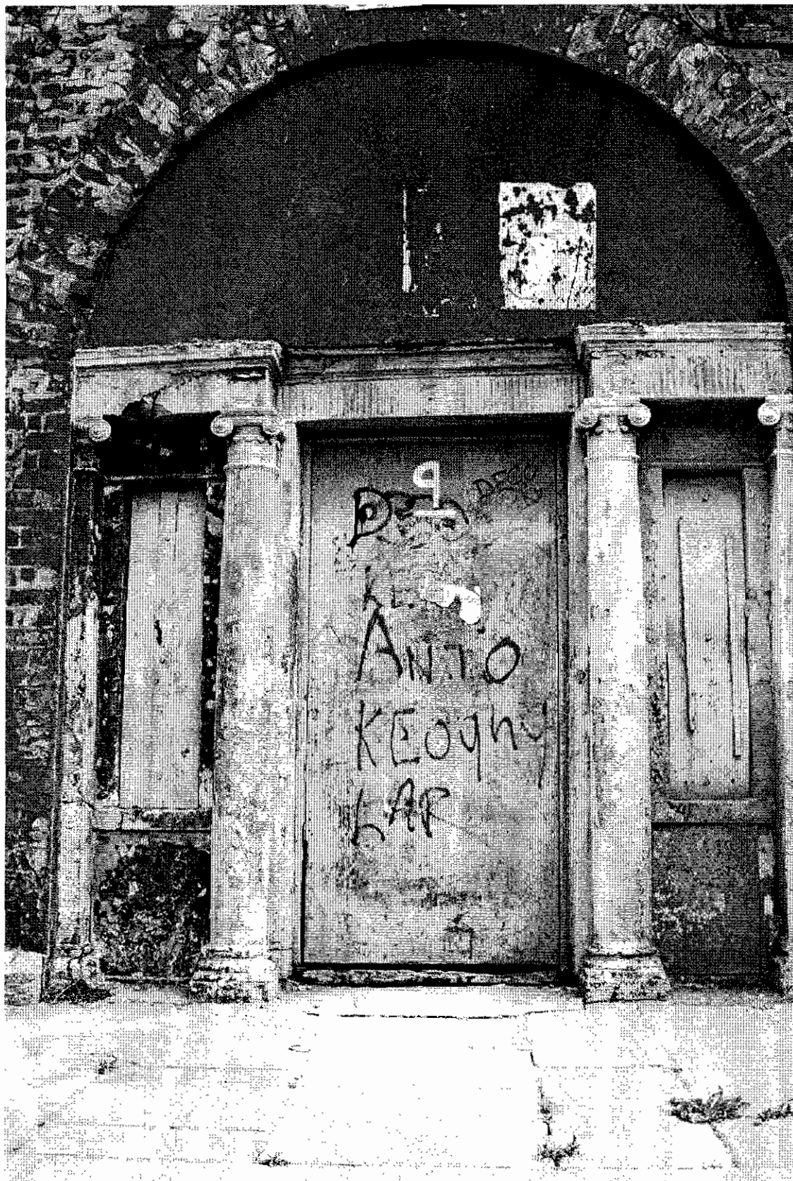
Figure 1: Dilapidated Georgian doorway adorned with the graffiti of contemporary Dublin. Photograph by Anne Maree Barry.
