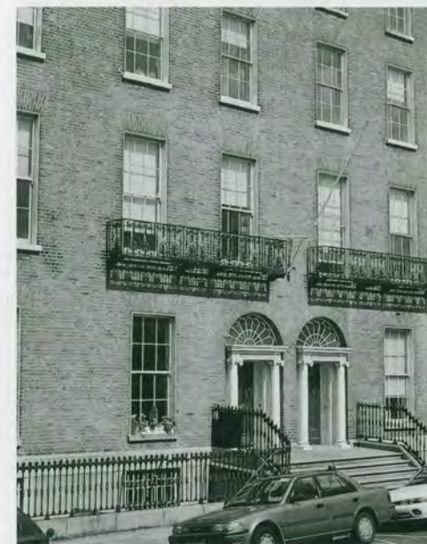
DIT Fitzwilliam House (Central Office).
