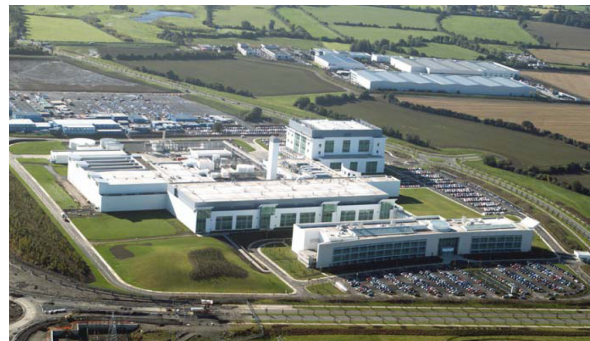
Figure 1 The Wyeth Biopharma Campus at Grangeecastle
