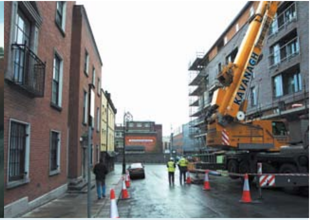
Fig.4.2.4 View towards Bolton Street from Henrietta Street
