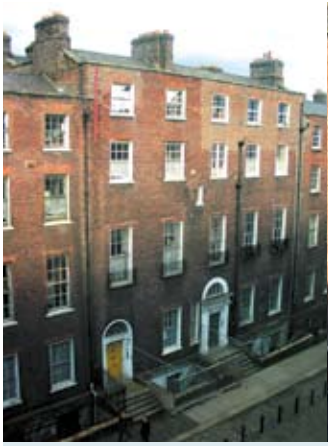
Fig.4.2.2 Pair of houses on north side of Henrietta Street
