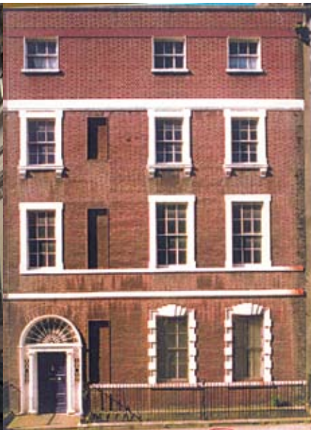
Fig.5.3.19 No.11, elevation, photo taken prior to commencement of current conservation work, from HARP/DCT Inventory
