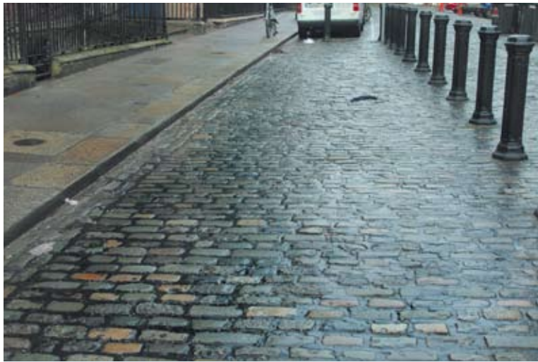
Fig.6.5.1 Detail of granite setts
