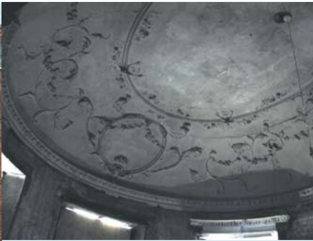
Fig.5.3.2 No.3, coved, bowed ceiling with rococo plasterwork
