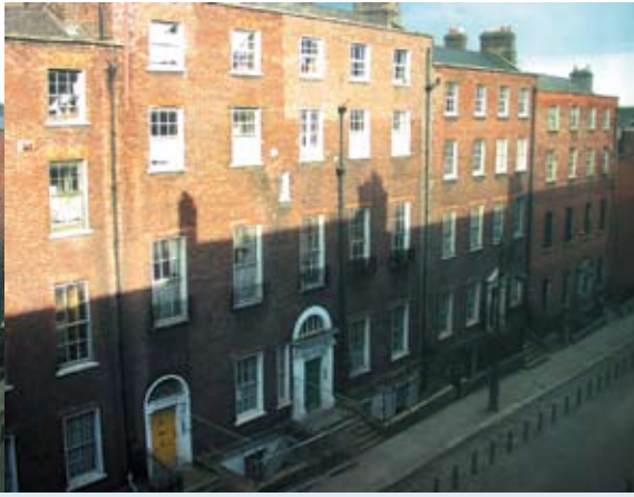
Fig.4.2.3 Terrace on north side of Henrietta Street
