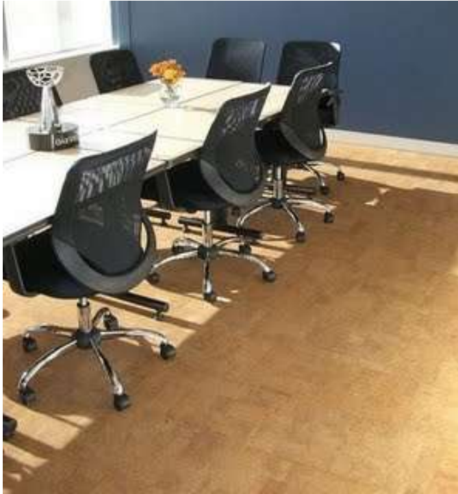
Fig. 11: Cork flooring in an office environment, where noise reduction is essential
