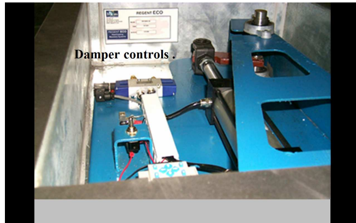
Figure 16. Reverse Flow Heat Recovery Damper
