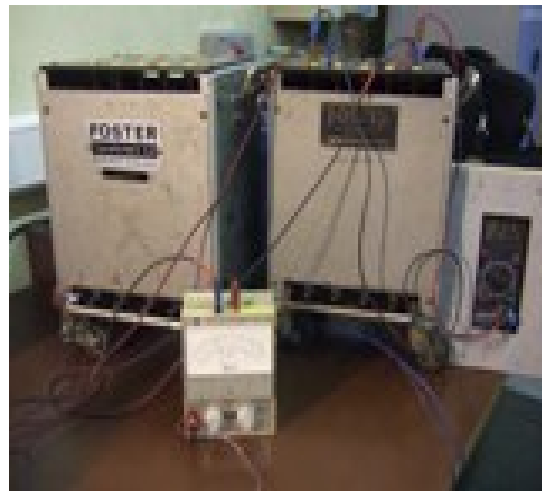
Figure 23. Transformer temperature monitoring
