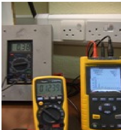
Figure 19. Neutral Current measurement for a 3 phase balanced CFL load
