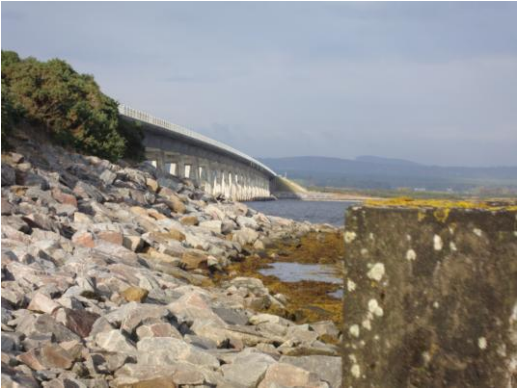
Figure 4 - Shows the location of the pier stem (right hand side of the picture) near the Dornoch bridge, Scotland
