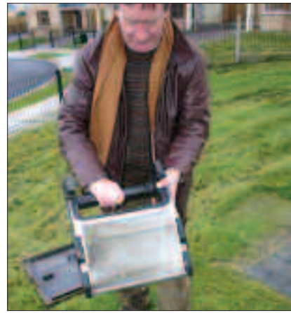
Fig. 2.5 Inline filter installed prior to rainwater entry to tank.
