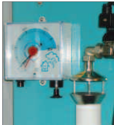
Fig. 2.8 Pressure meter showing level of rainwater in storage tank.
