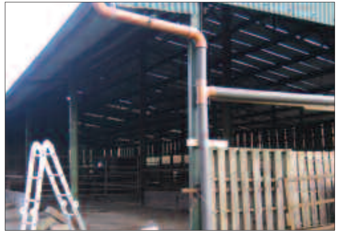
Fig. 3.12 Installation of regime 2.
