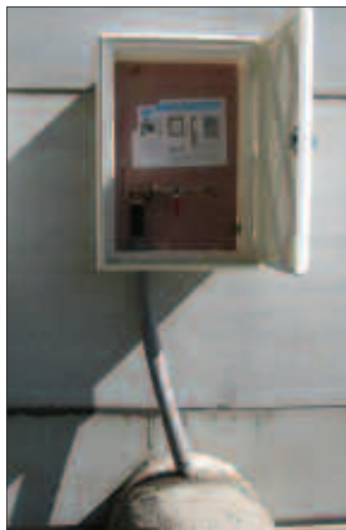
Fig. 3.8a&b Rainwater reservoir water quality sampling points.
