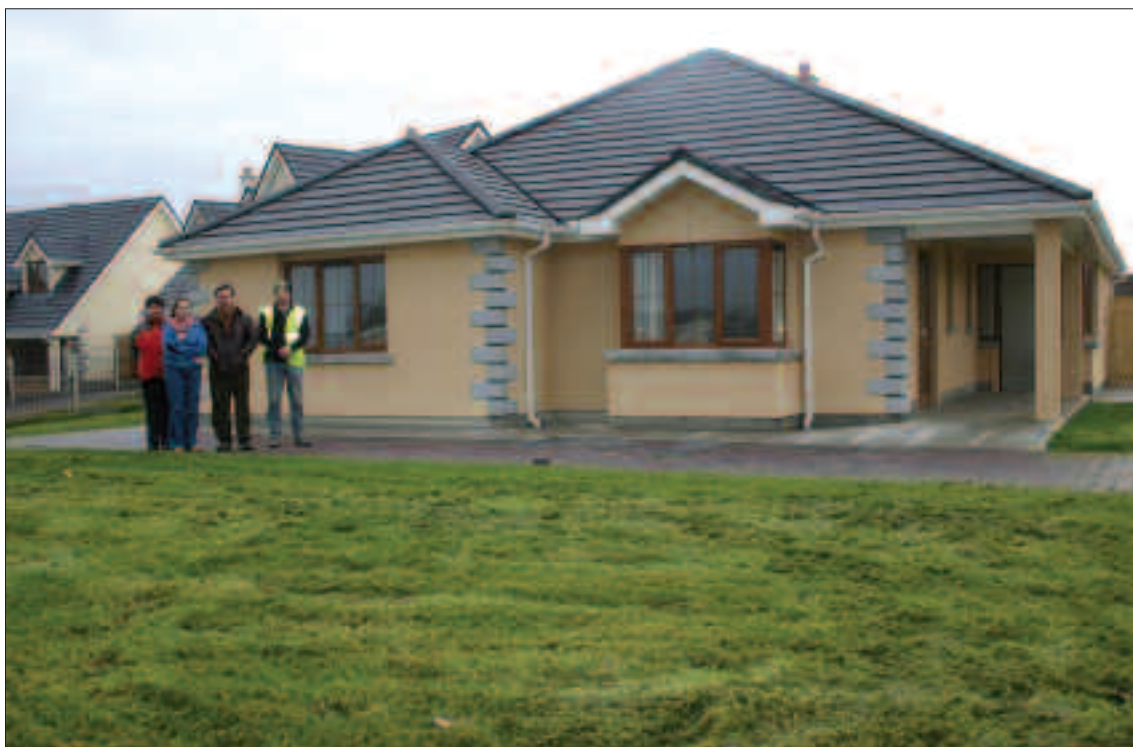
Fig. 2.21 The house at Ballinabrannagh, County Carlow in which the rainwater harvesting system was installed.
