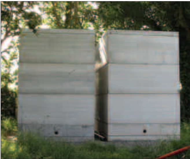
Fig. 3.5 Rainwater storage reservoir.
