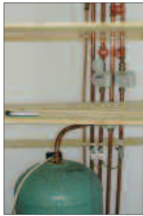
Fig. 2.11 & 2.12 Water meters in the hot press.
