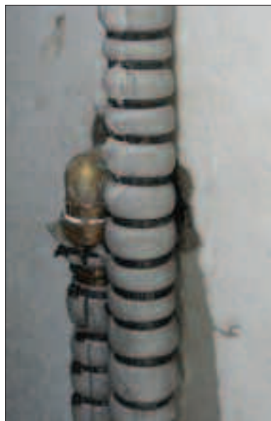
Fig. 3.7a & b Mains water top-up system.
