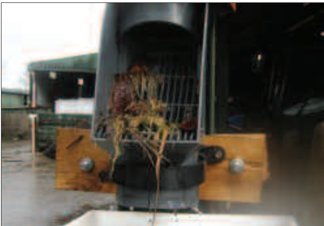
Fig. 3.13 and Fig. 3.14 A Lindab leafbeater™ and a BRAE™ filter installed.
