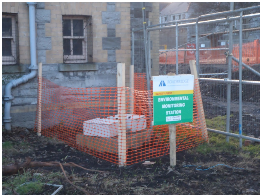
Monitoring Station No 2 @ Mortuary Building
