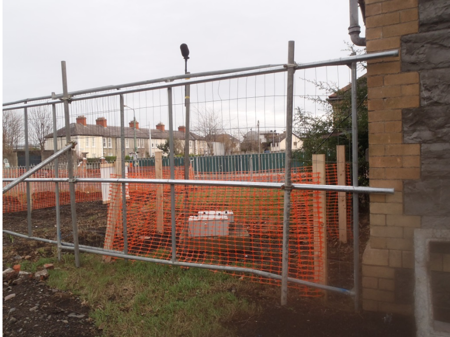
Monitoring Station No 2 @ Mortuary Building
