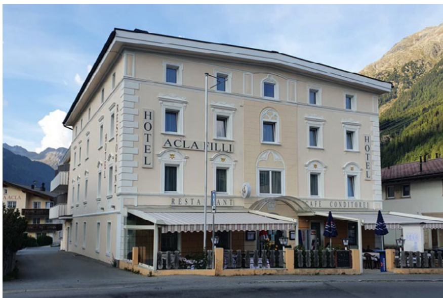
Fig.14: Renovated Building ready for connection to the district heating system
