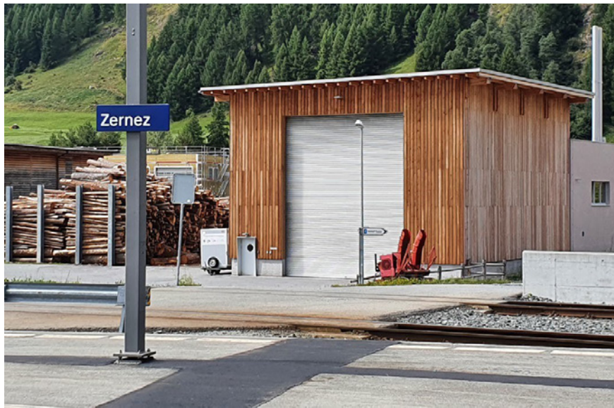
Fig.13: New woodchip district heating plant
