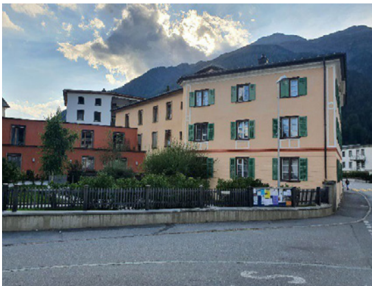
Fig.1: Back-yard of pilot building “Röven 8” F
