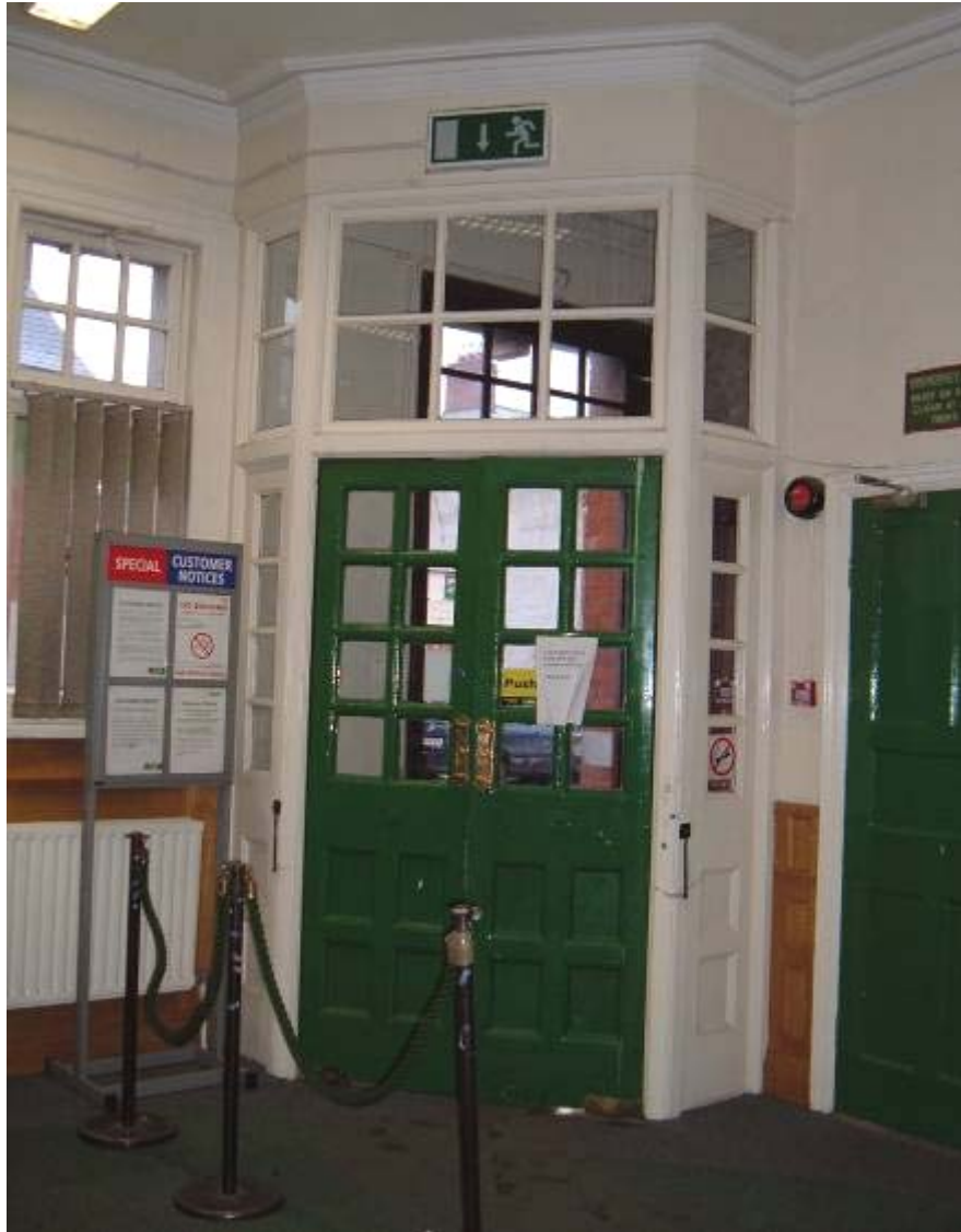
Figure 6/49 – Kells P.O., 1902; Original Glazed Screen to Public Office; Photo, Author 2007
