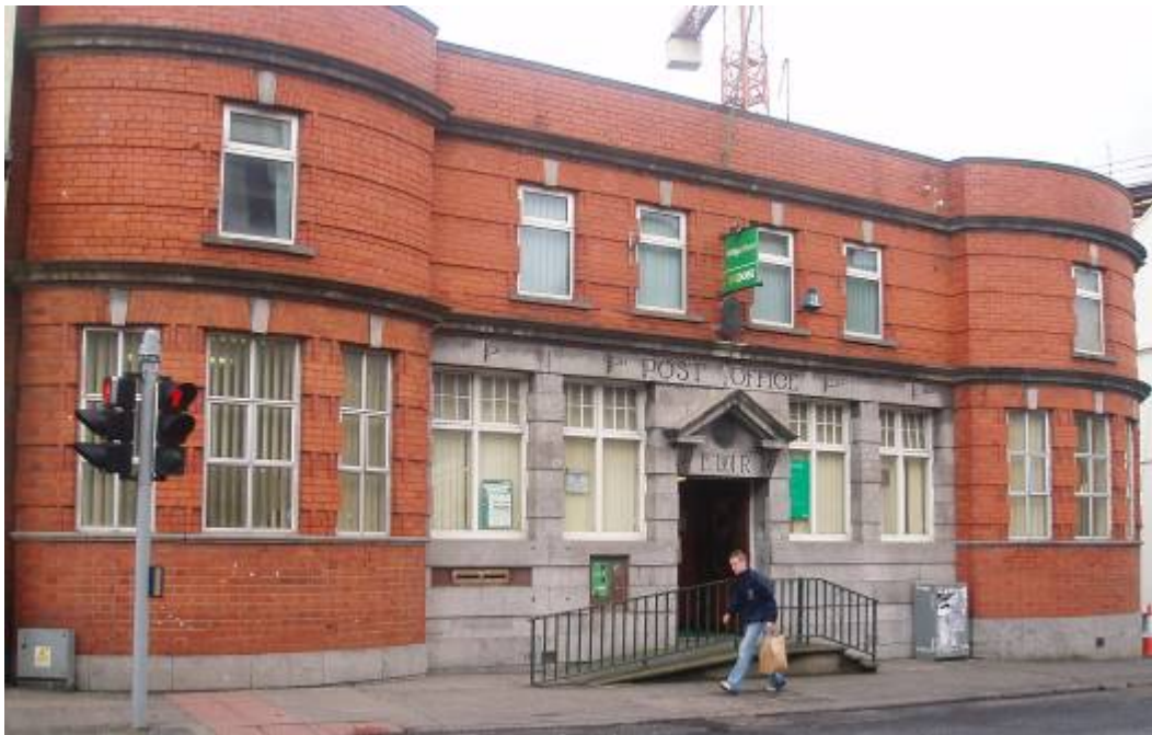
Figure 5/32 – Sligo P.O., c.1899; Brick and Stone Post Office; Photo, Bernadette Solon, 2006
