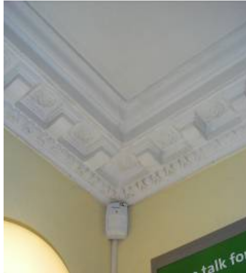
Figure 7/64 – Ballsbridge P.O., c.1915; Existing Coving Detail; Photo, Author, 2007
