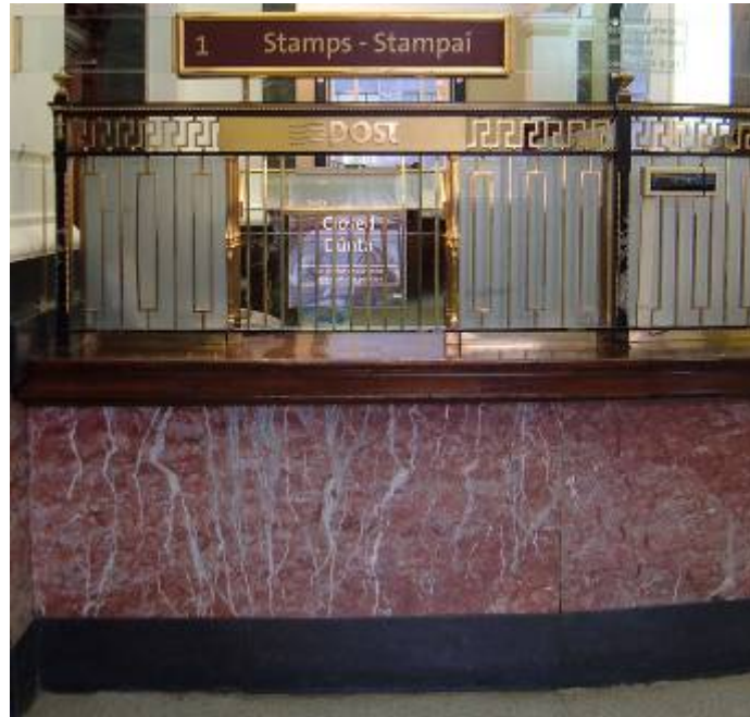
Figure 8/73 – G.P.O., Dublin; Detail of Public Counter and Screen; Photo, Author, 2007
