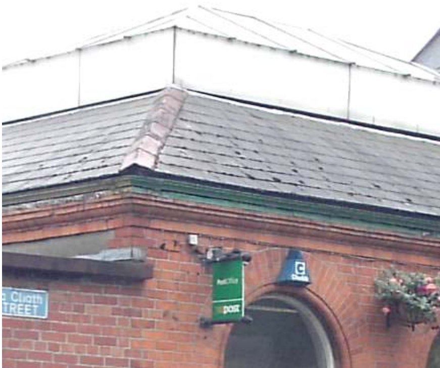
Figure 5/90 – Kildare P.O., c. 1910; Photo showing eaves brick detailing; Photo, Author, 2006
