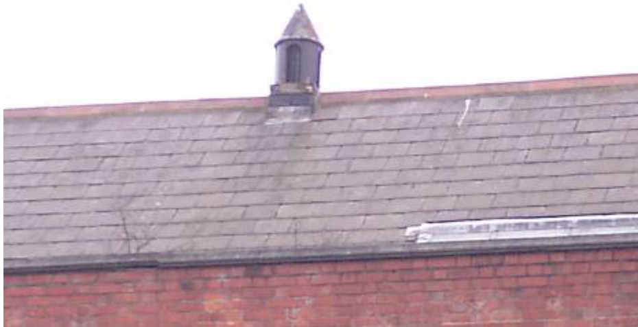
Figure 7/60 – Ballsbridge P.O., c.1915; Roof Ventilator, Photo, Author 2007
