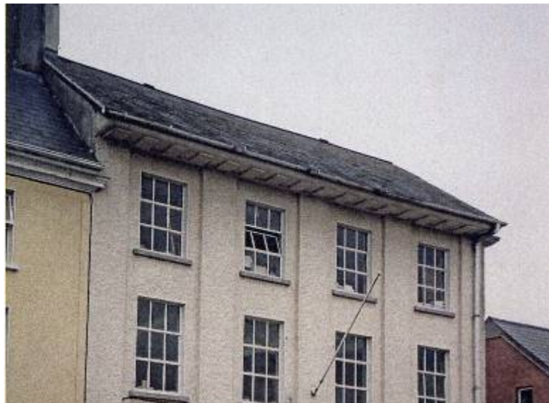
Figure 6/44 - Tullamore P.O., c.1908; Eaves Detail; Photo, Caroline Pegum, OPW
