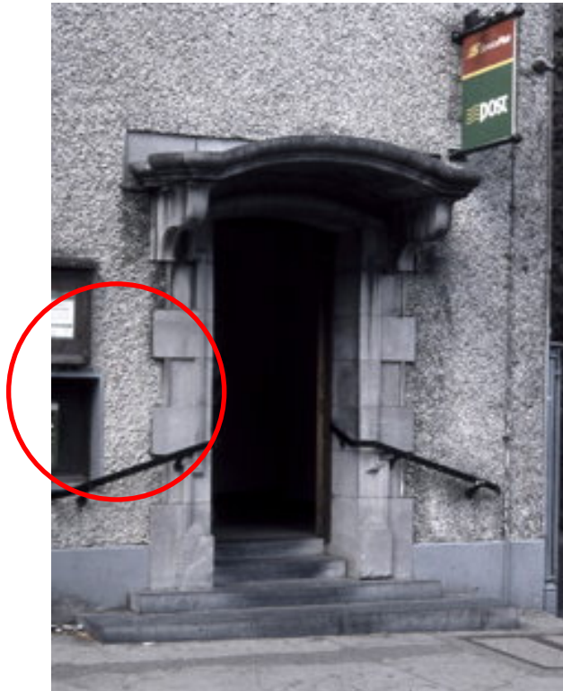
Figure 8/74 – Athy P.O.; Photo showing the period stamp dispenser units. Photo, courtesy NAIH Buildings of Ireland , 2003
