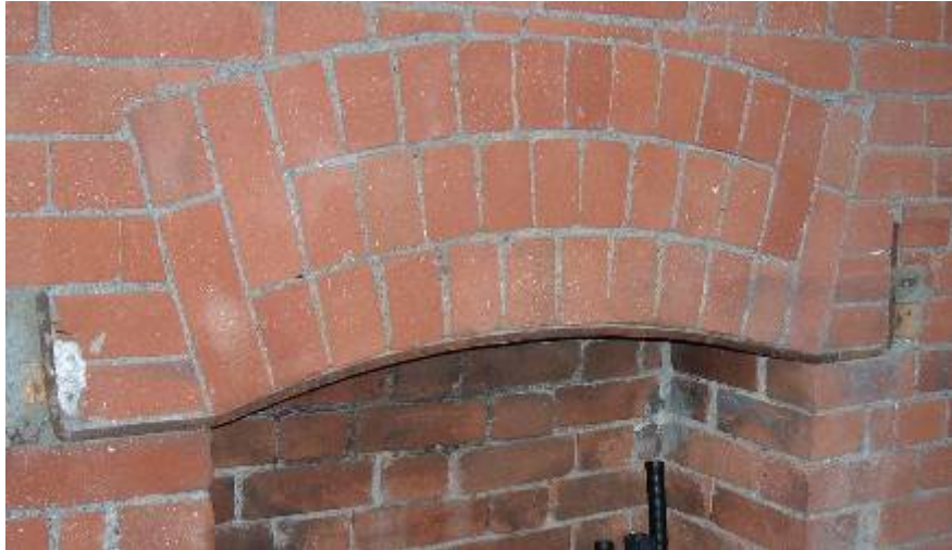
Figure 7/56 – Rathmines P.O., c.1883; Original arch to fireplace; Photo, Author, Feb 2007
