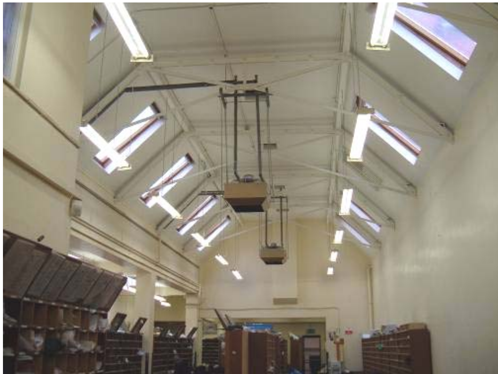
Figure 6/48 – James's Street Post Office; Sorting Room, Original Roof Structure, Photo; Author, 2006
