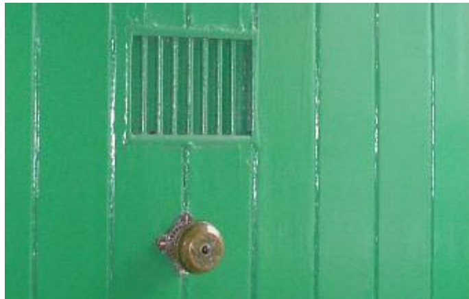
Figure 7/61 – Ballsbridge P.O., c. 1915; Door Grille Detail, Original Entrance Door, Photo, Author, 2006
