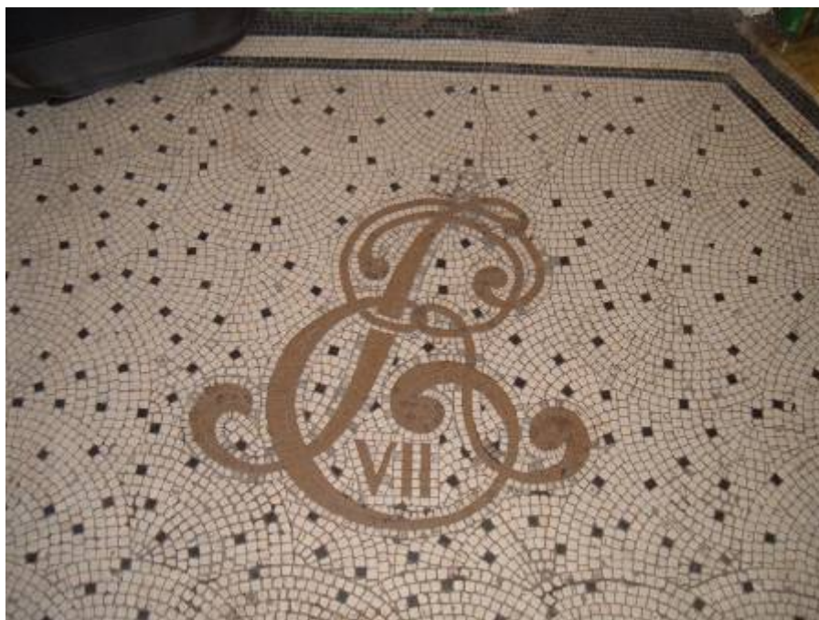
Figure 5/47 – Kells P.O., Royal Insignia inlaid in Entrance Porch Floor; Photo, Author, 2007
