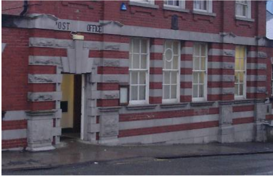
Figure 5/85 – Castlebar P.O., 1902; Decorative Stonework on Front Façade; Photo, Author 2005
