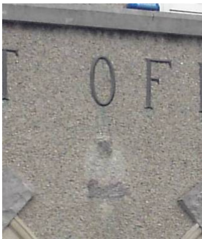
Figure 7/87 – Westport P.O., c. 1900; Repair work on Front Façade; Photo, Author, 2007
