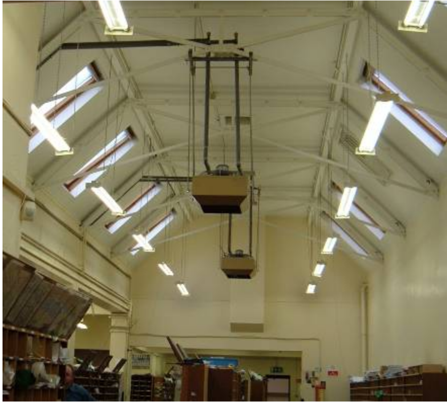
Figure 7/39 – James's Street Former P.O.; Sorting Office Roof Structure; Photo, Author, 2006
