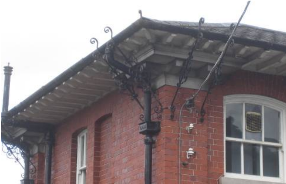
Figure 5/89 – Castlebar P.O., 1902; Decorative eaves brackets; Photo, Emer Crean, 2007
