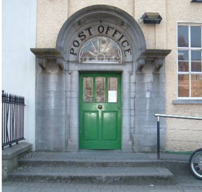
Figure 6/43 - - Tullamore P.O., c.1908; Doorcase Detail; Photo, Author 2007
