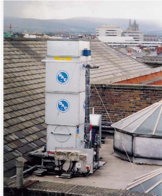
**Figure 4.** General view of forced draft counter-flow cooling tower. Overall dimensions 0.914 x 1.207 x 3.436 high excluding air intake. (local marshalling terminals for data monitoring and control system shown at low level)
