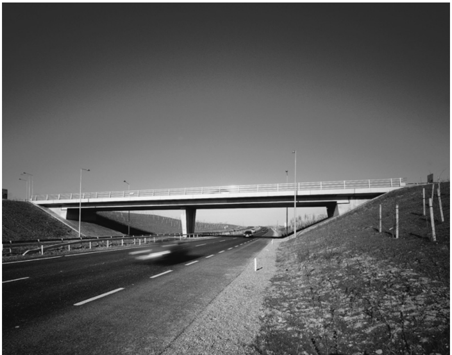
Figure 1.2 Bridge on Arklow bypass, Ireland (Source: Arup. Photographer: Studioworks).
